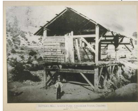
Sutter's Mill in 1848 (Bancroft Library, UC Berkeley)
